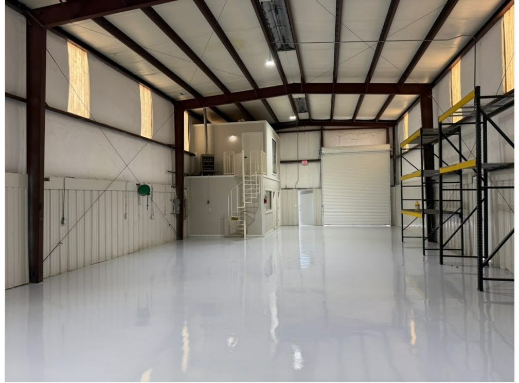
Inside of Warehouse
