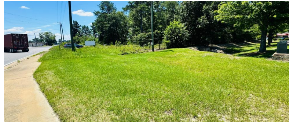
Sidewalk Along Firetower Road
