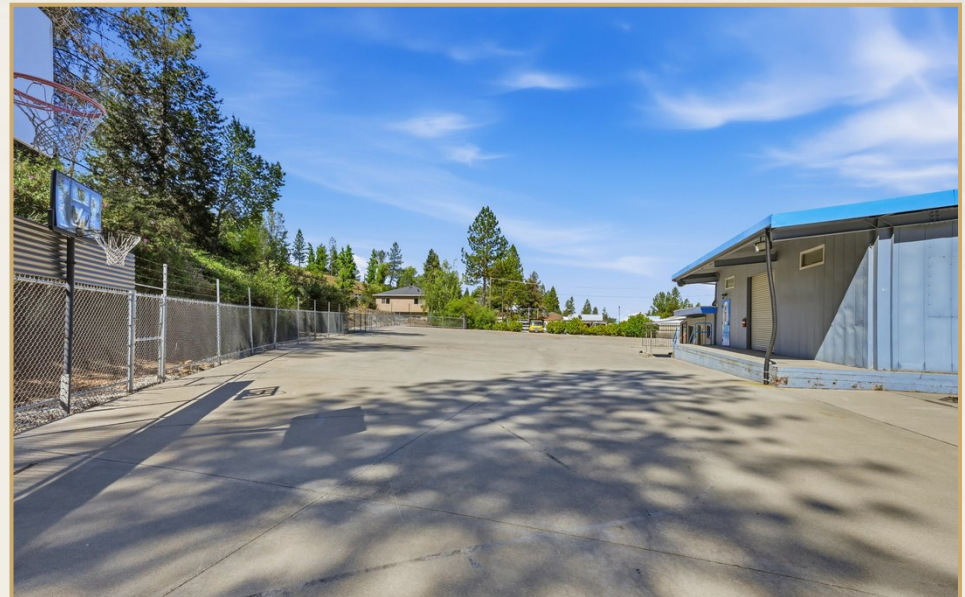
Dock-High Loading + Concrete Yard
