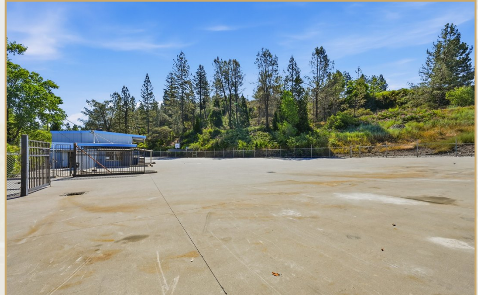
Fully-Fenced Concrete Yard
