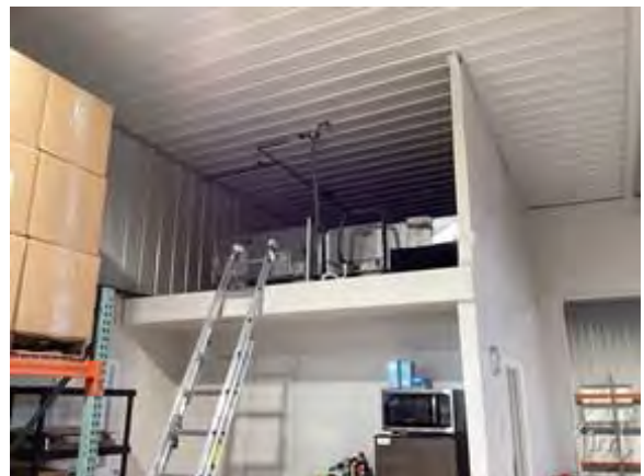
Interior view of subject property
