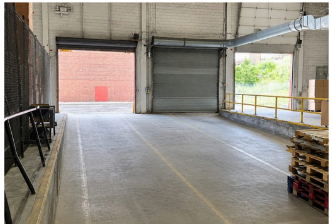
Interior loading — dock-height plus drive-in access.
