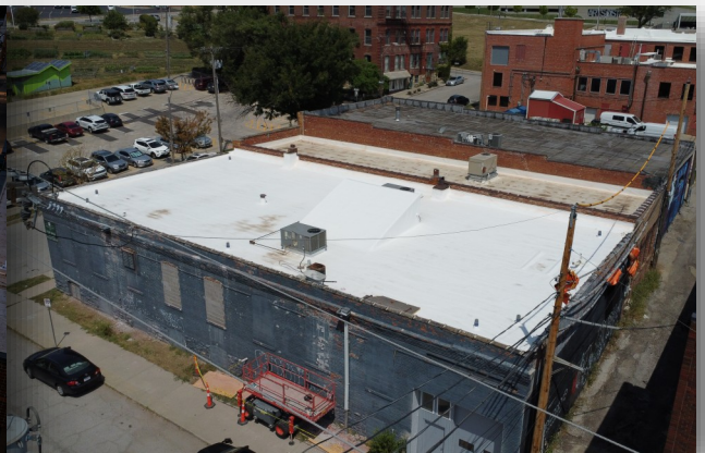
New roof installed July 2022
