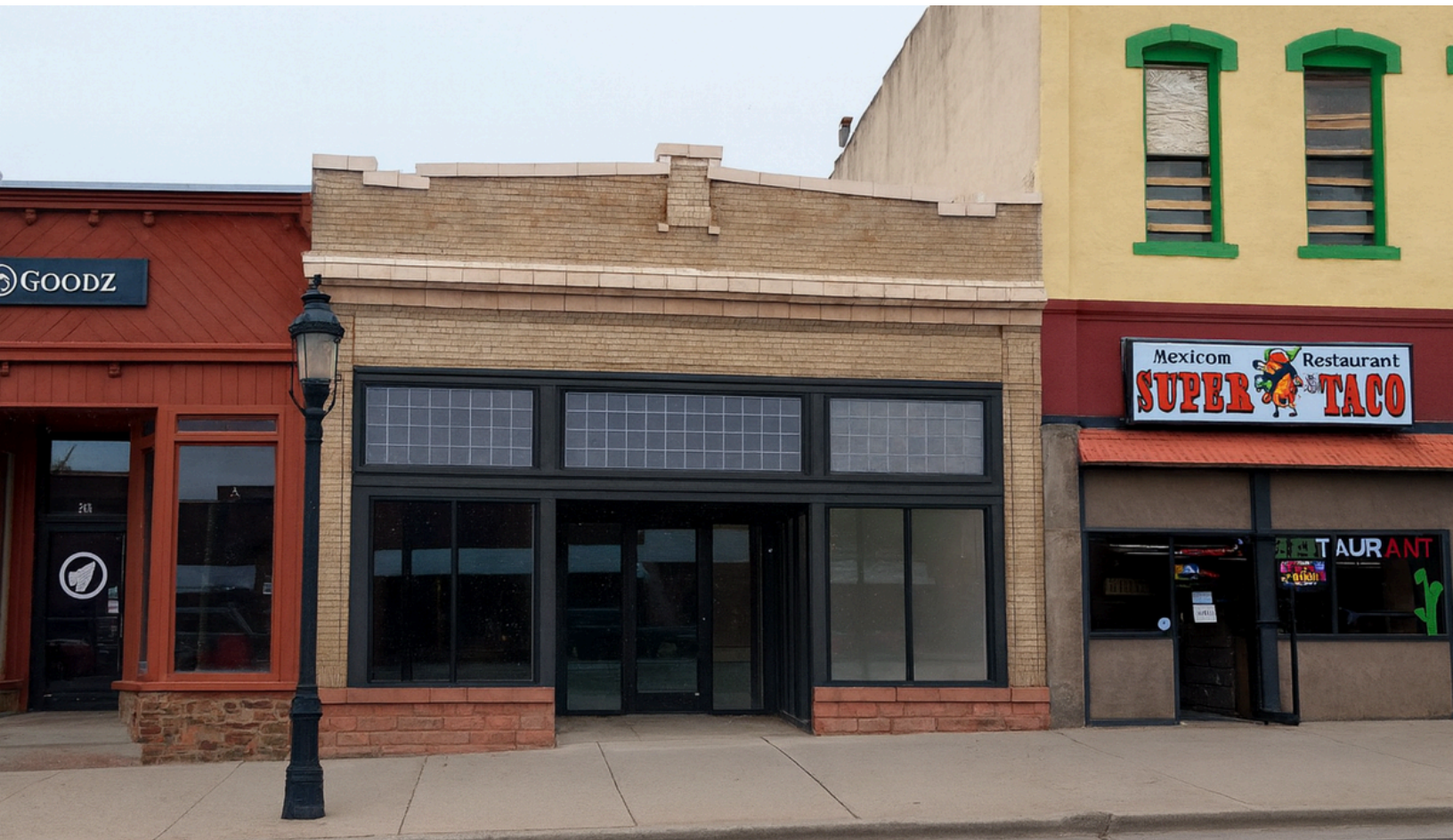
818 Grand Ave - Exterior of Dental / Medical Building (Front)
