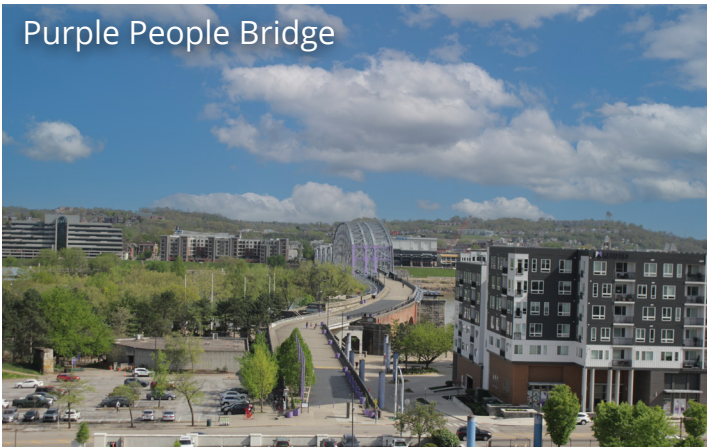
Scenic Rooftop View
