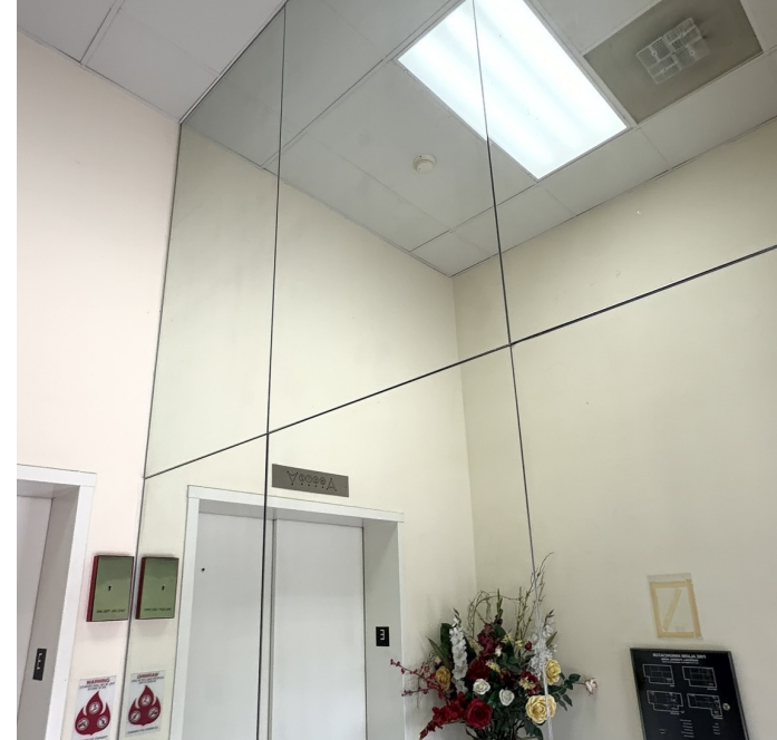
Elevator | ADA Accessibility
