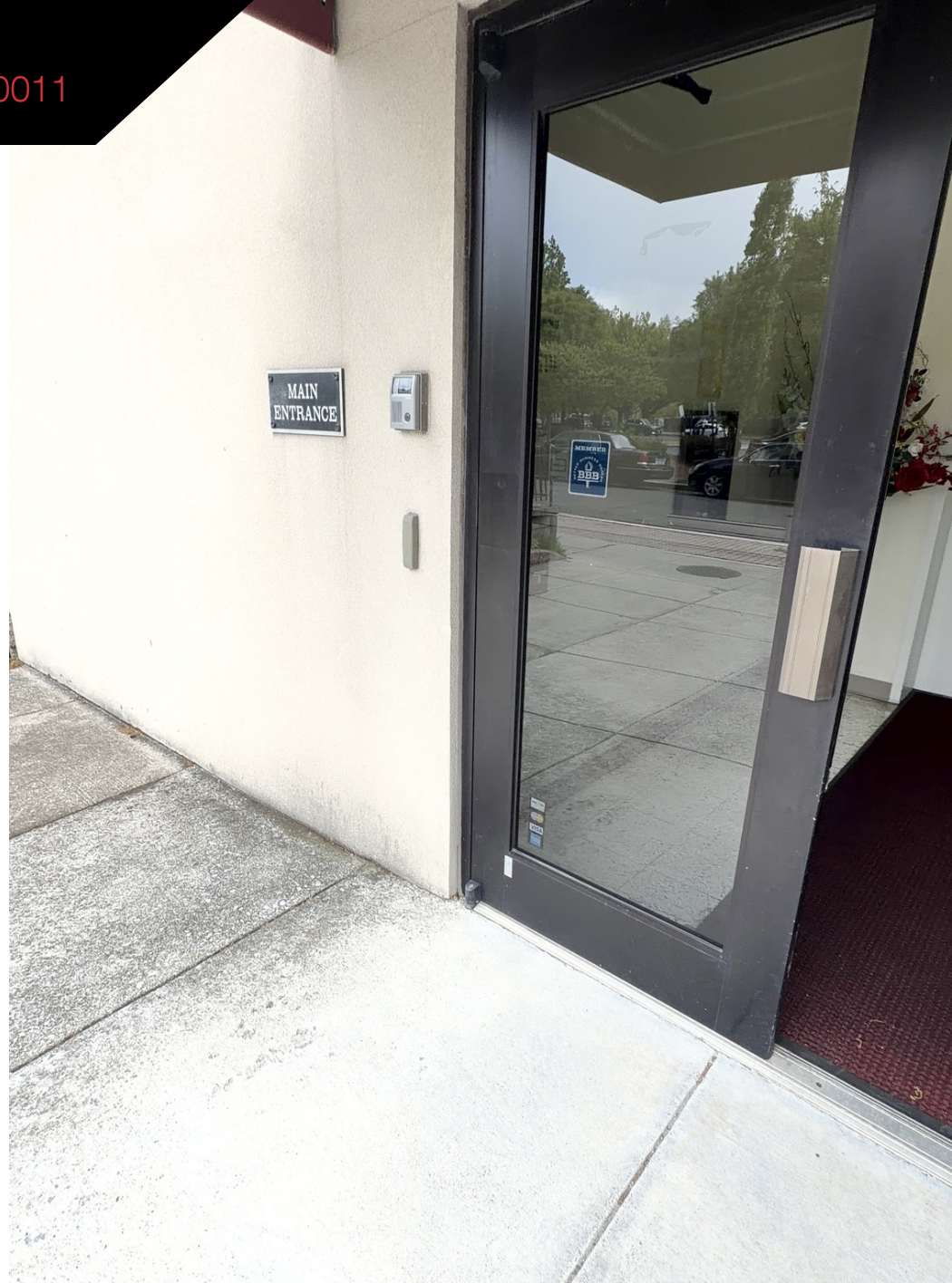
Main Entrance Door
