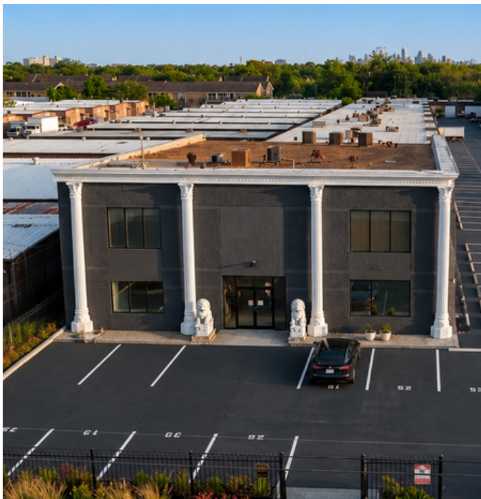
Front aerial view
