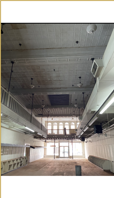
Ground Floor Interior — Tin Ceiling
