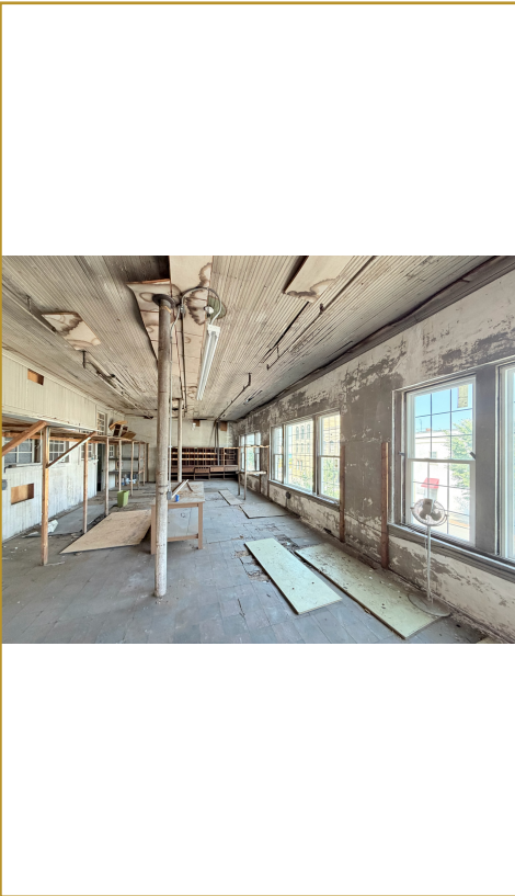
Upper Floor Interior — New Windows
