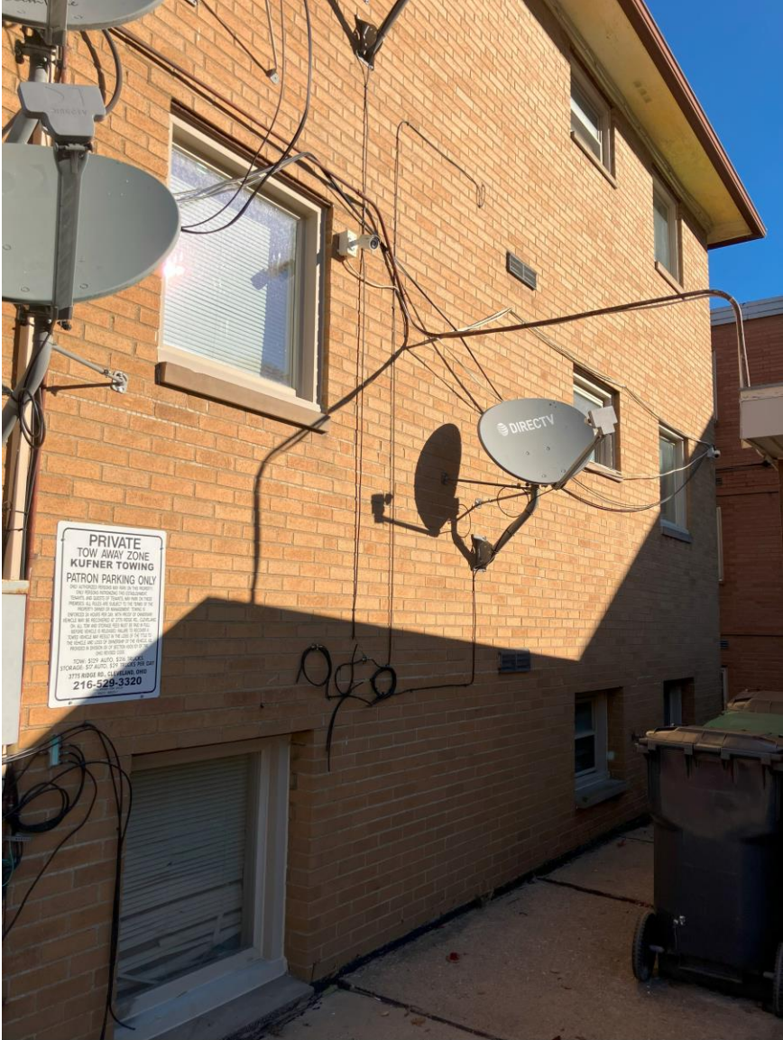
Looking northeast at the rear wall
