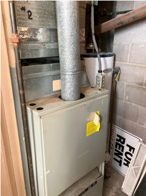
Typical furnaces and hot water tanks in mechanical closets
