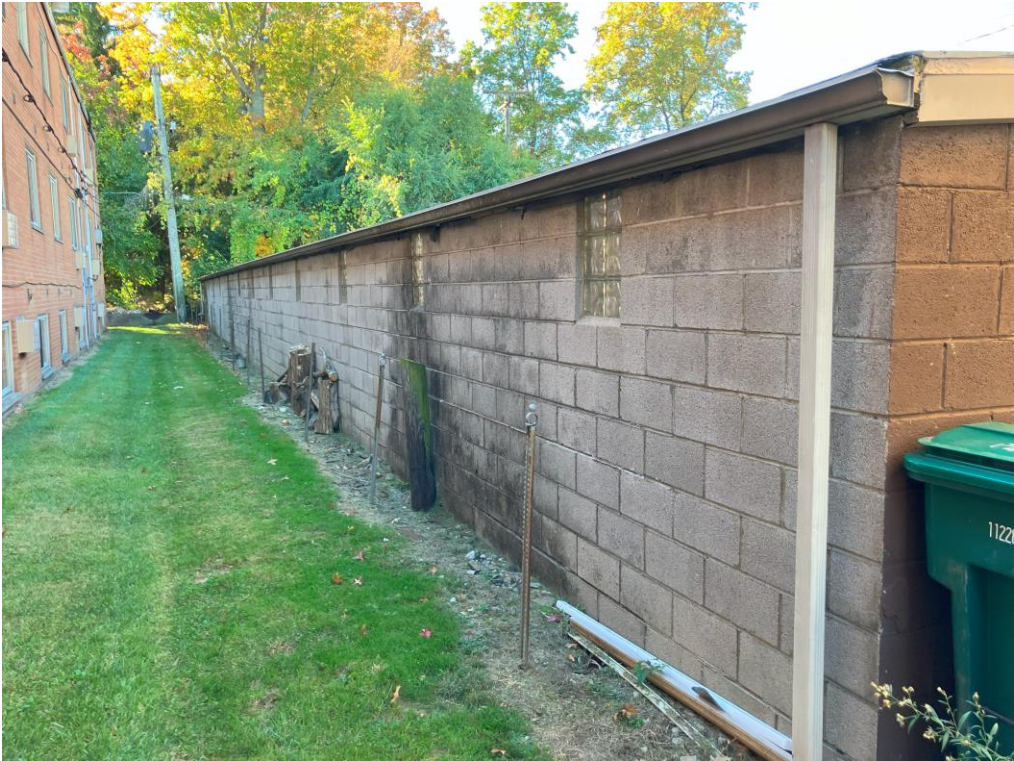
Looking south along rear garage wall
