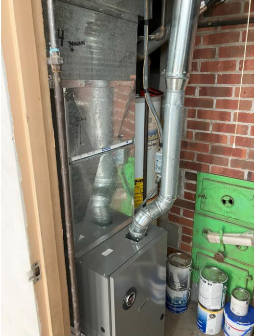
Typical furnaces and hot water tanks in mechanical closets
