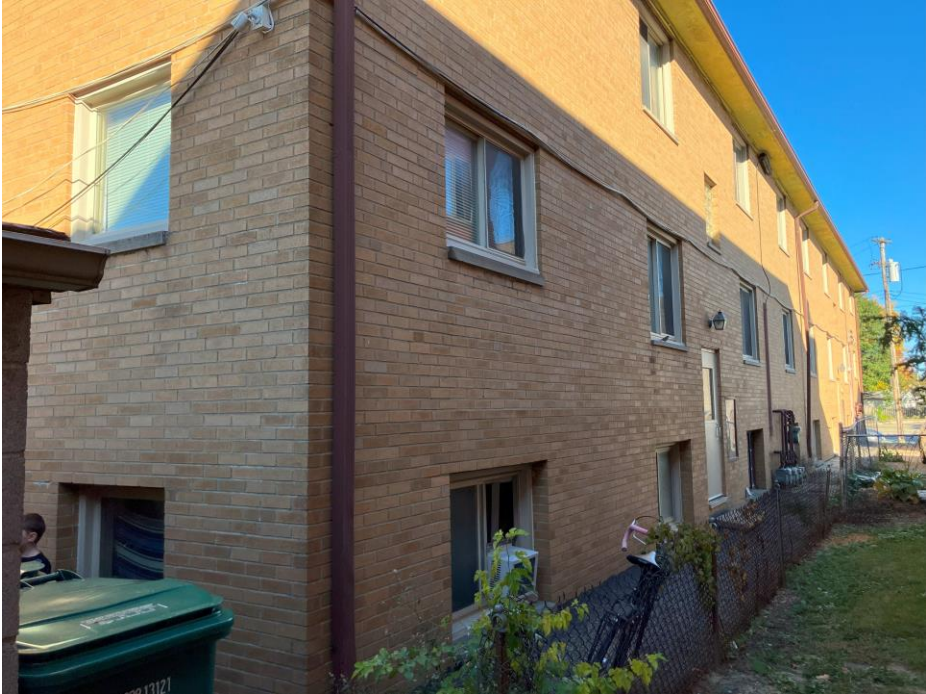
Looking northwest at left wall and rear of building.
