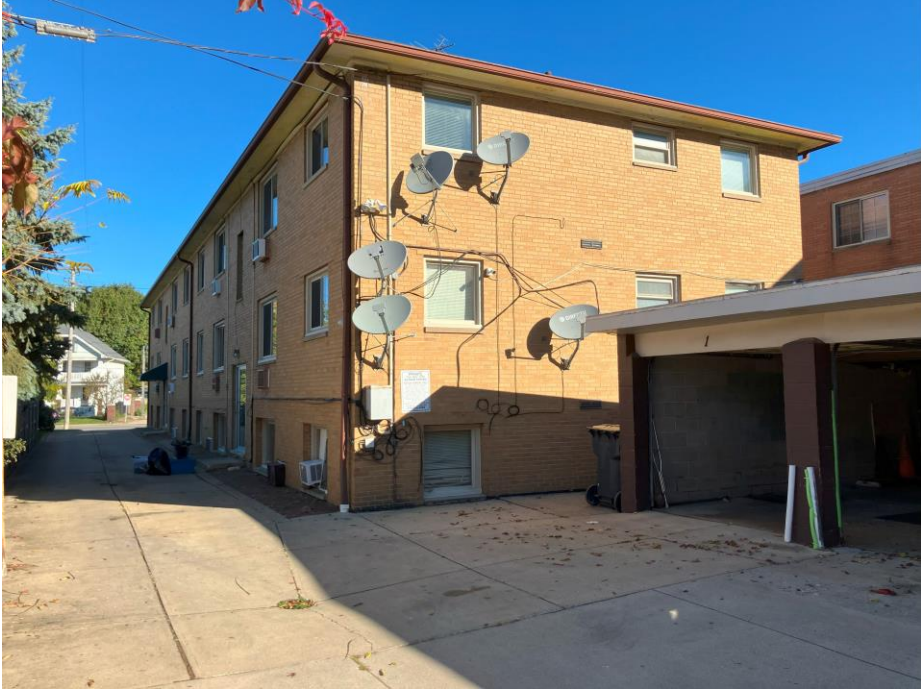
Looking northeast at the building rear and right sides
