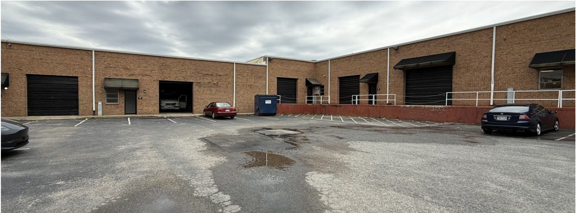
REAR OF THE BUILDING
