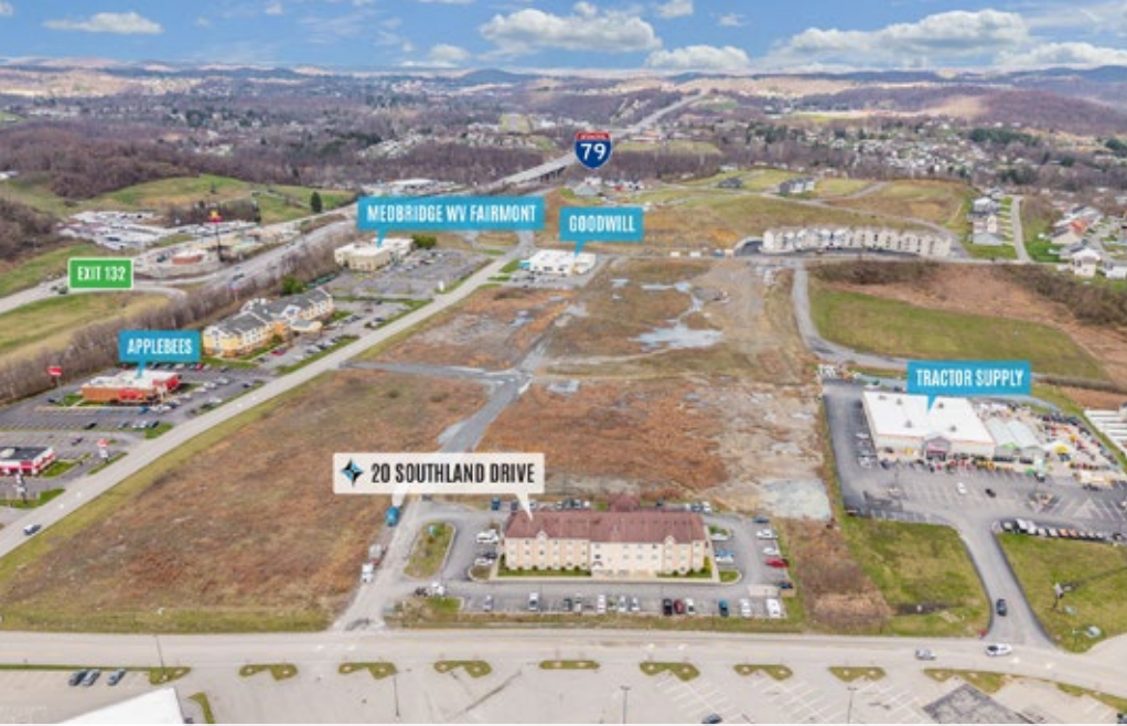
Aerial Facing Northeast.
