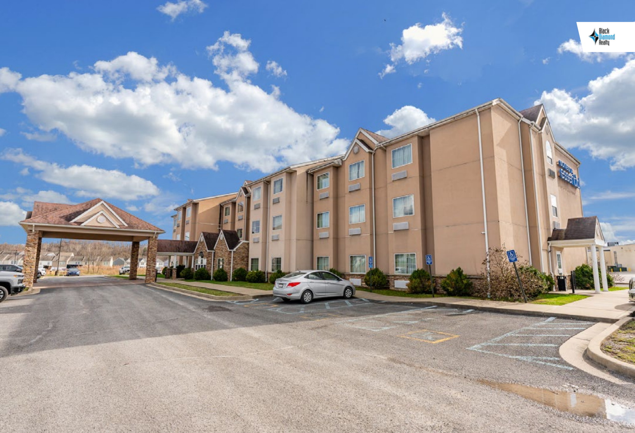
Parking Lot and Main Entrance.
