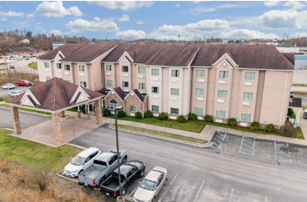
Aerial Facing South.
