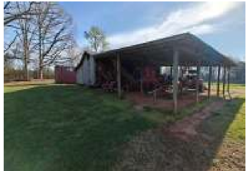
8) A shed on the northern-central portion of the site.
