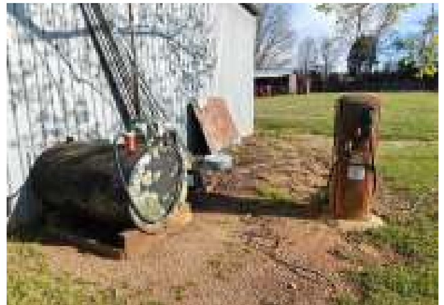
28) AST and dispenser pump observed beside the shed shown in Photograph 6.
