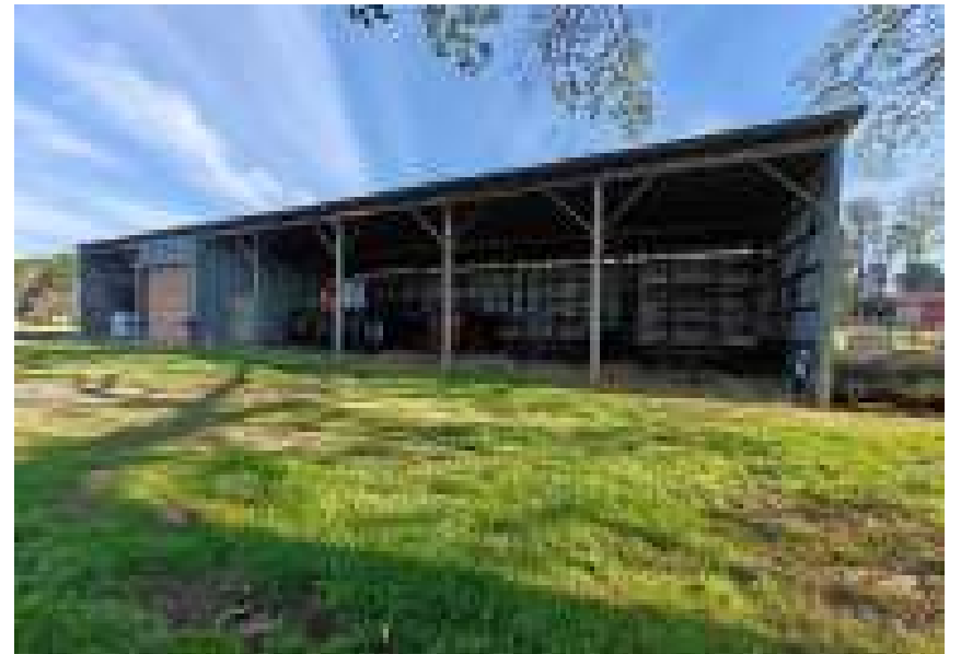
6) A shed on the northern-central portion of the site.
