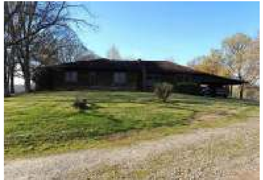
2) The back of the house that occupies the central portion of the site.
