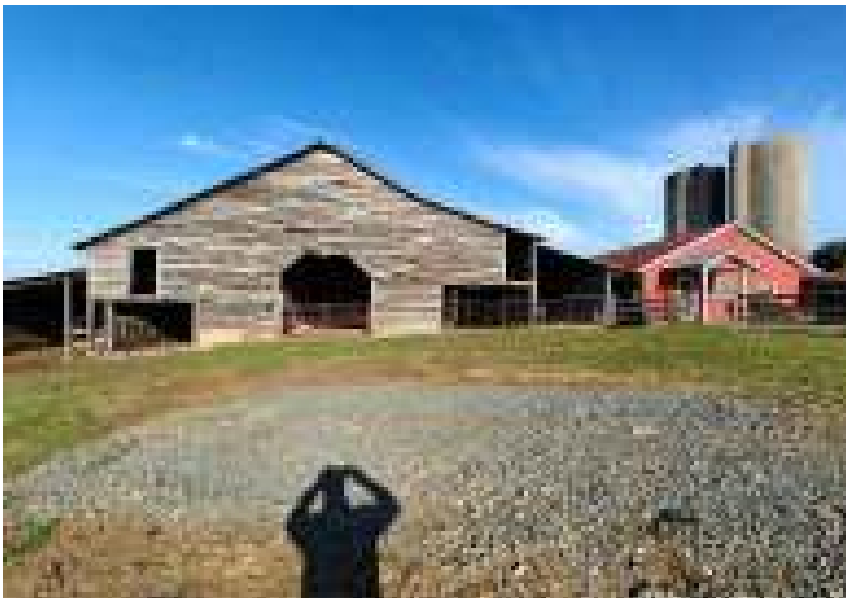
3) Barn and guesthouse on the southwestern portion of the site.
