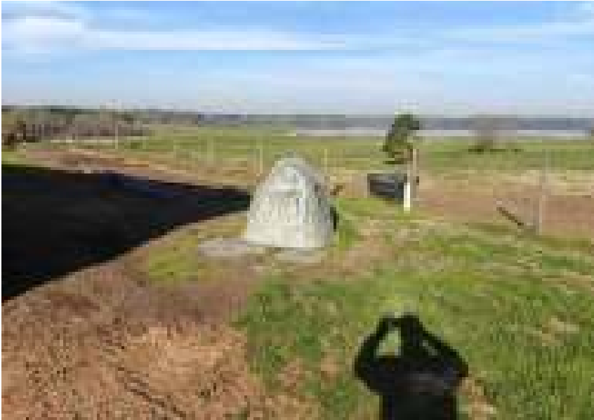
13) A water supply well observed on the central portion of the site.
