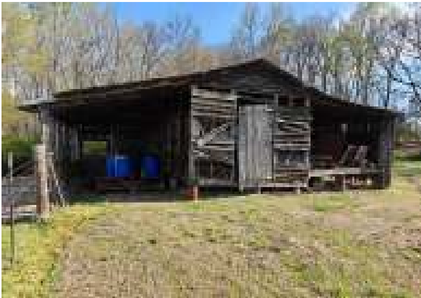
7) A shed on the northern-central portion of the site.
