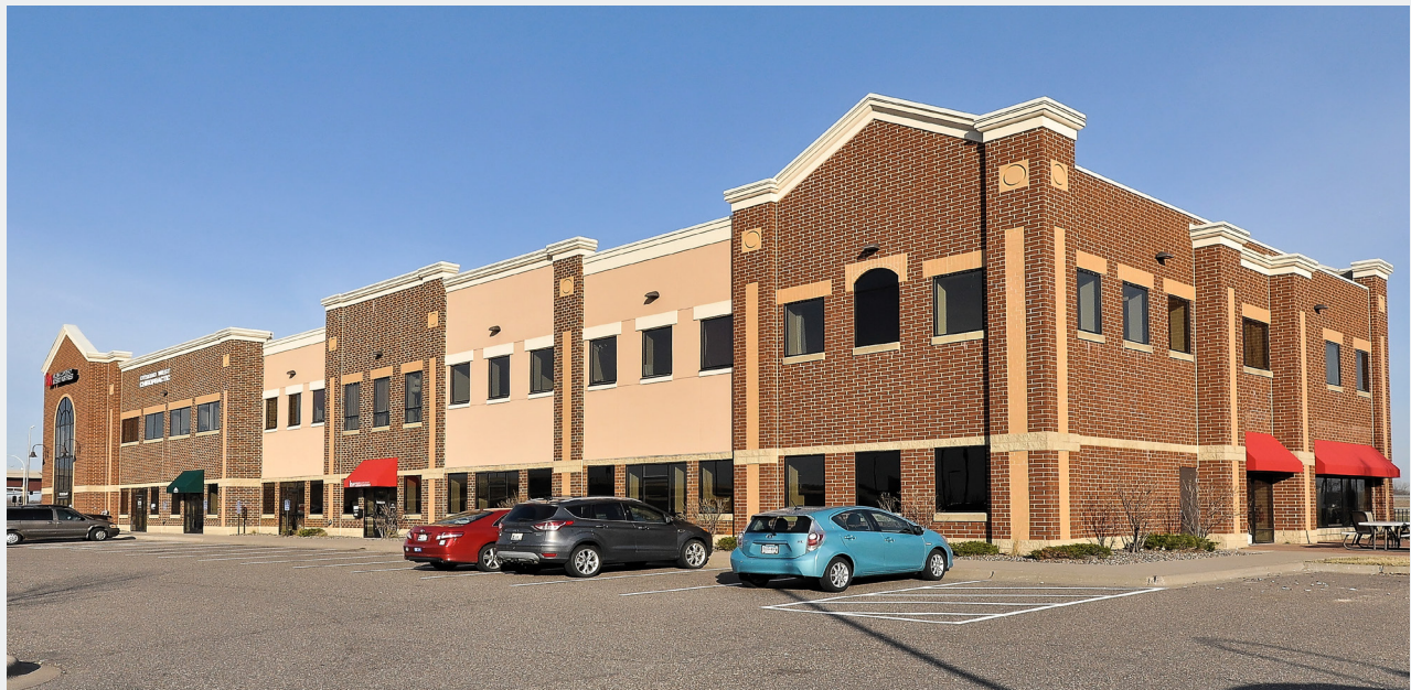
Back of Building
