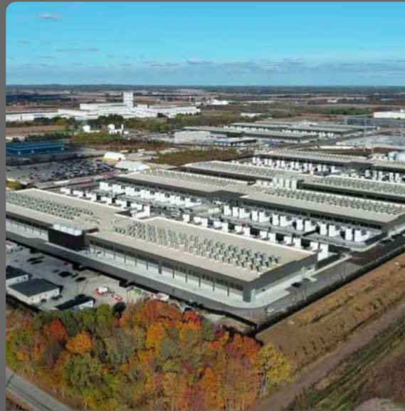
Amazon Data Center
