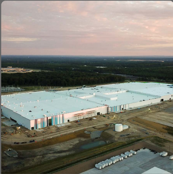
GM Samsung EV Battery Plant
