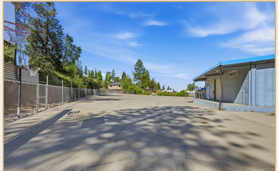
Dock-High Loading + Concrete Yard
