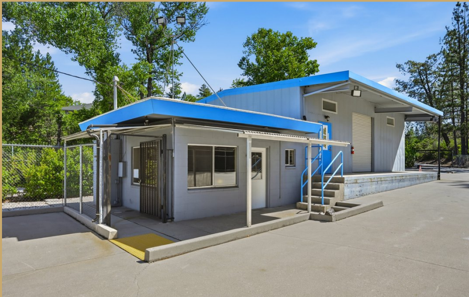
Renovated Shop & Office
