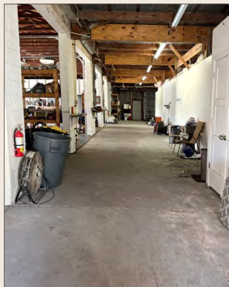
Main Warehouse Area
