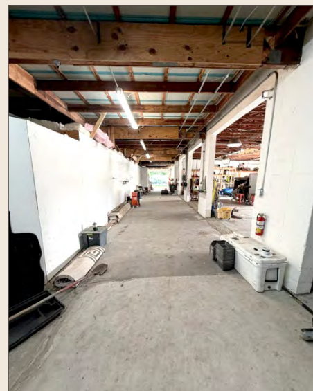
Main Warehouse Area
