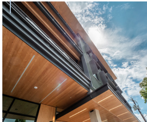
MASS TIMBER CONSTRUCTION
