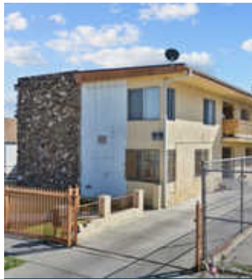
1036 West 95th Street, Los Angeles, CA 90044
