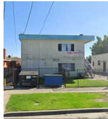
820 West 95th Street, Los Angeles, CA 90044
