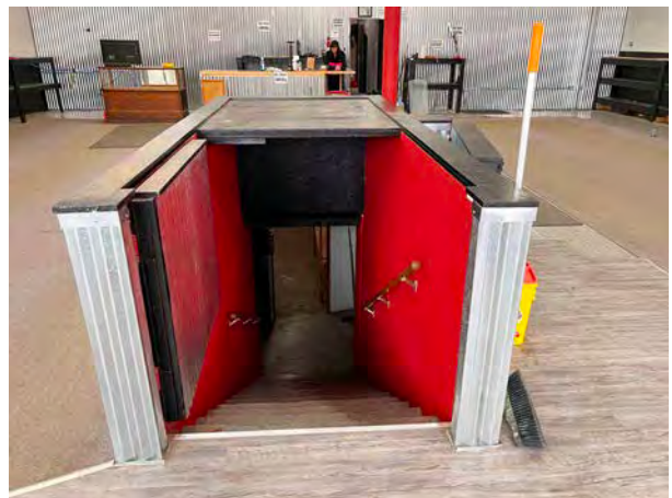
Main Level - Stairs to Lower Level
