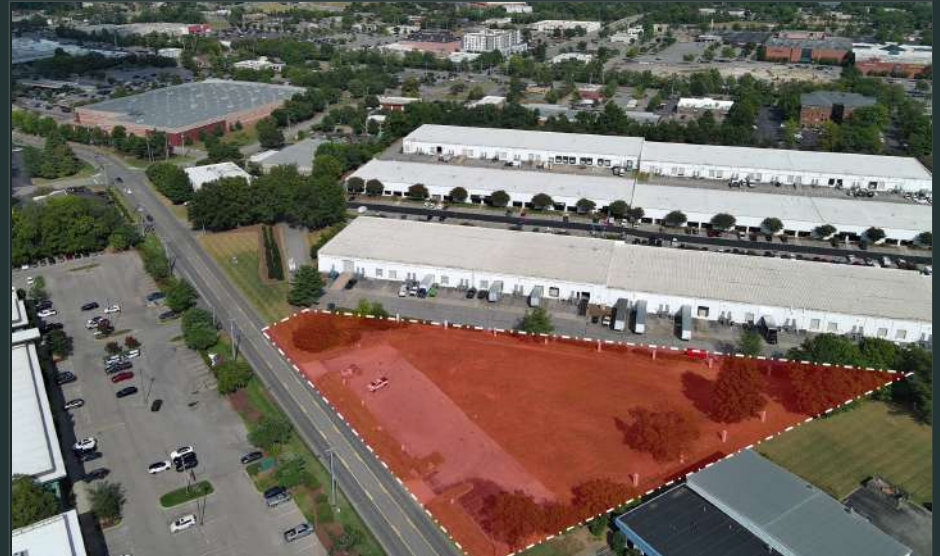
SITE — SIDE FACING
