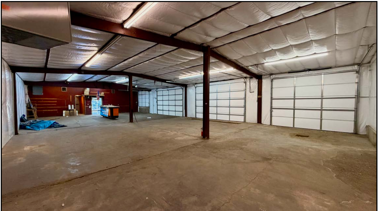
Heated warehouse · overhead doors & dock
