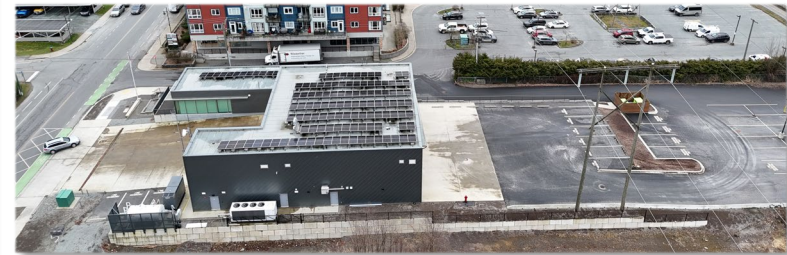
View looking South New Firehall (parking under power lines)
