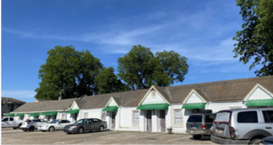
Main guestroom building frontage
