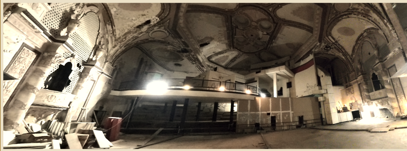
The auditorium and former balcony beneath the vaulted plaster ceiling
