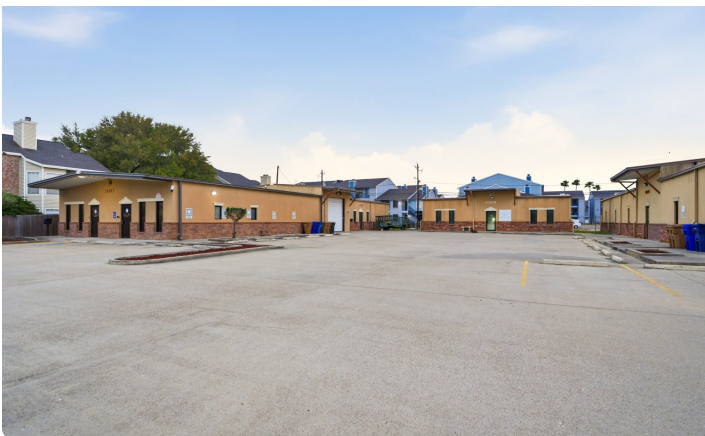
Front Building Elevation — Suites A & B (left) & Suite C (middle)
