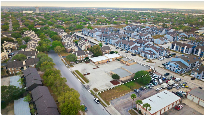
Aerial — Southwest View with Property Boundary
