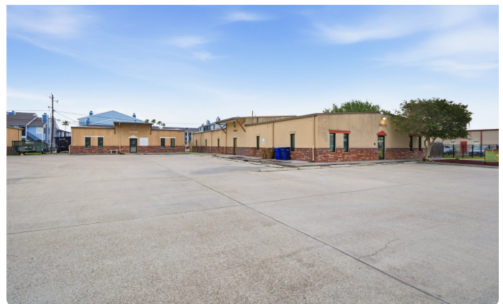
Front Building Elevation — Suite C (middle) & Suite D (right)
