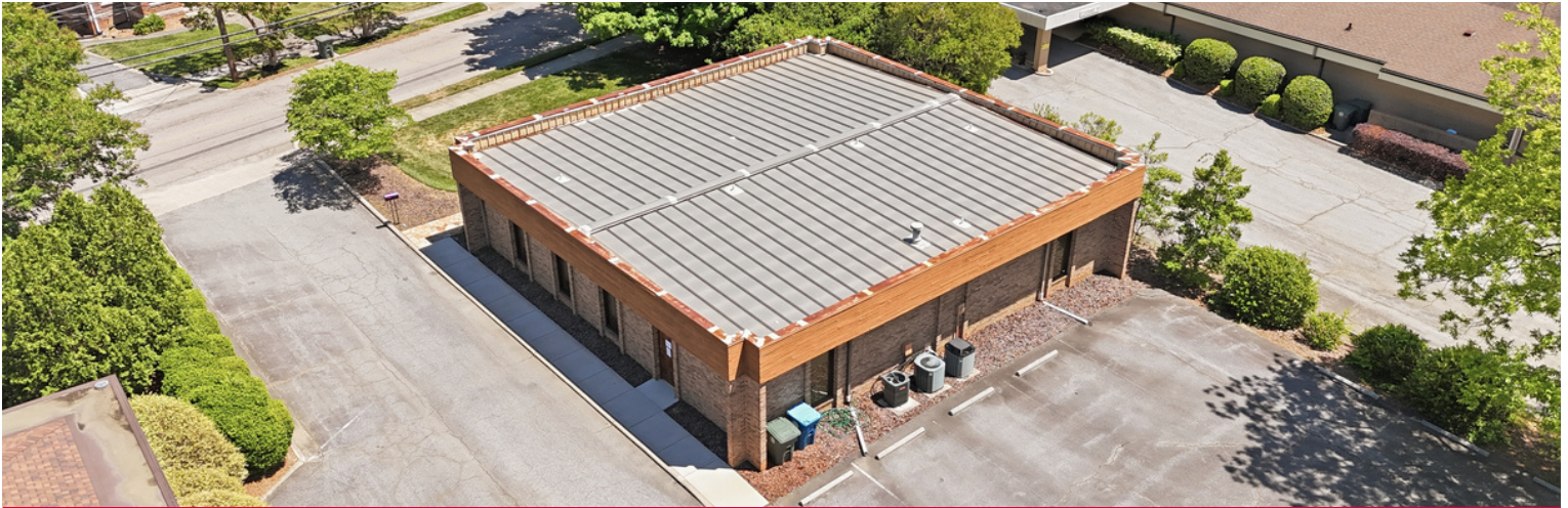
Aerial view looking north — Novant Health Rowan Medical Center visible top-right
