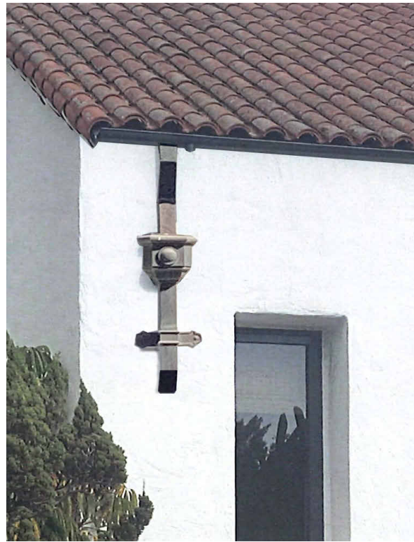
RECESSED WINDOWS AND RAINWATER SCUPPER COLLECTOR
