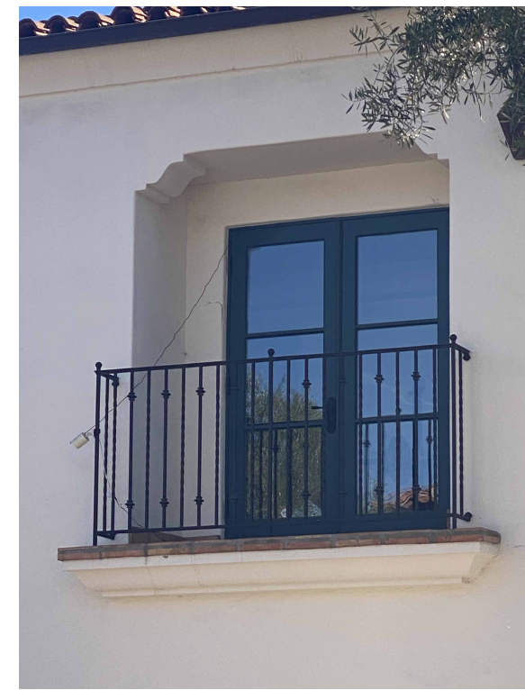
RECESSED BALCONY AND IRON GUARD RAIL
