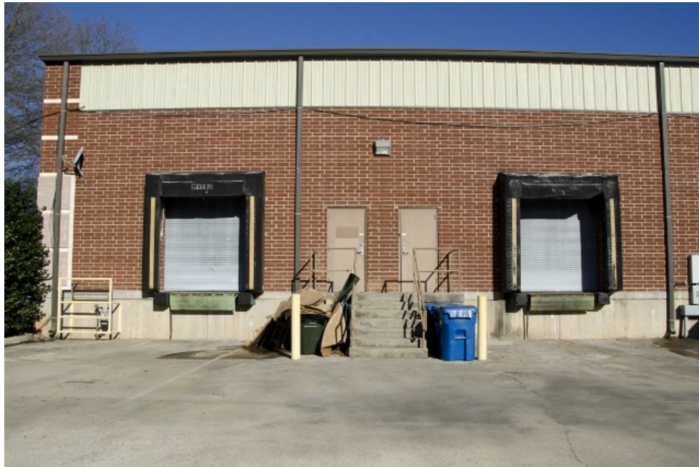
Dock / overhead doors
