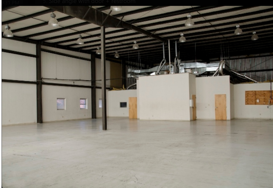
Warehouse bay · Unit H warehouse package
