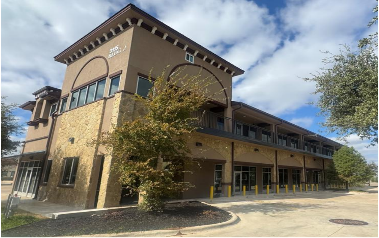
Figure 2: South East Elevation
