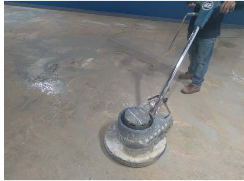
New polished concrete throughout facility
