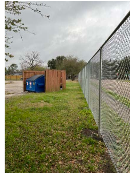
New perimeter fencing
