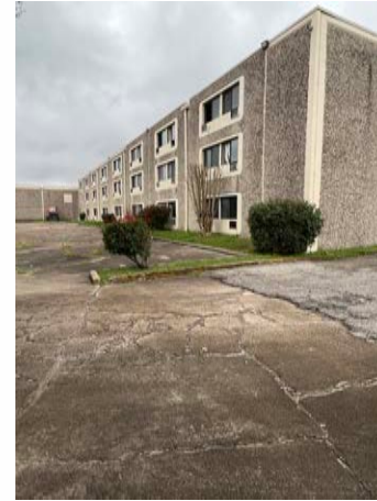
New exterior paint & LED security lighting
