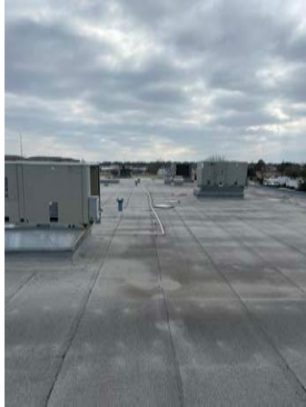
Updated HVAC and Roof
