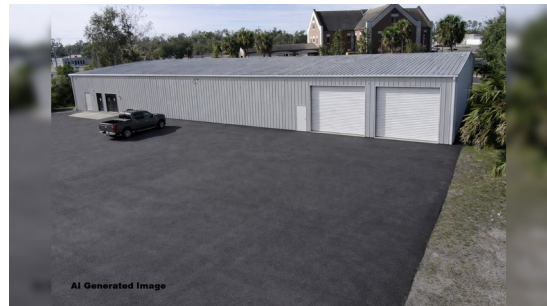
Preview concept rendering of a potential light industrial / warehouse conversion. See the following page for an enlarged illustrative concept.
