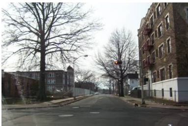
Lower Main Street Redevelopment Area
