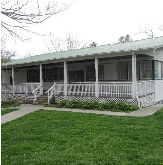
Front of Second Building Looking East
