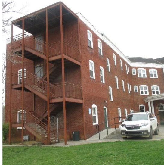
Rear of Primary Looking Southeast
