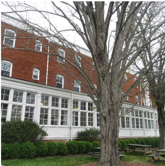
Rear of Primary Looking Southwest
