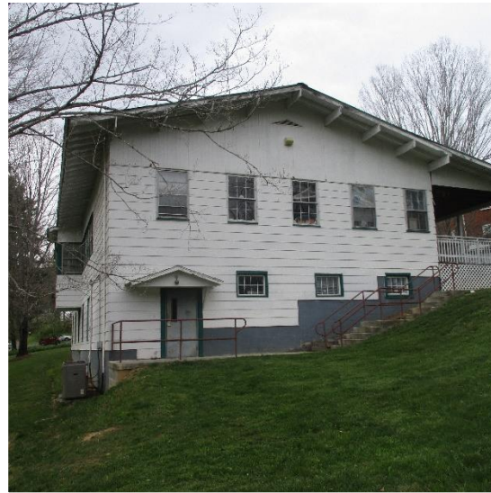
Rear of Second Building Looking West
