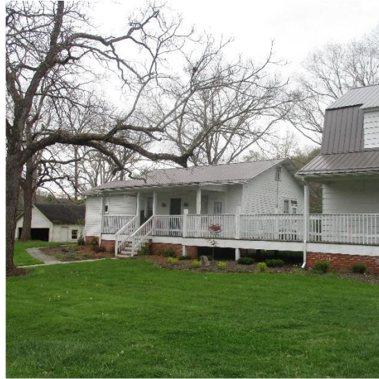
3rd Structure Looking West (Attached)
