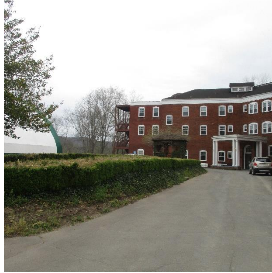
Rear of Primary Looking Southeast
