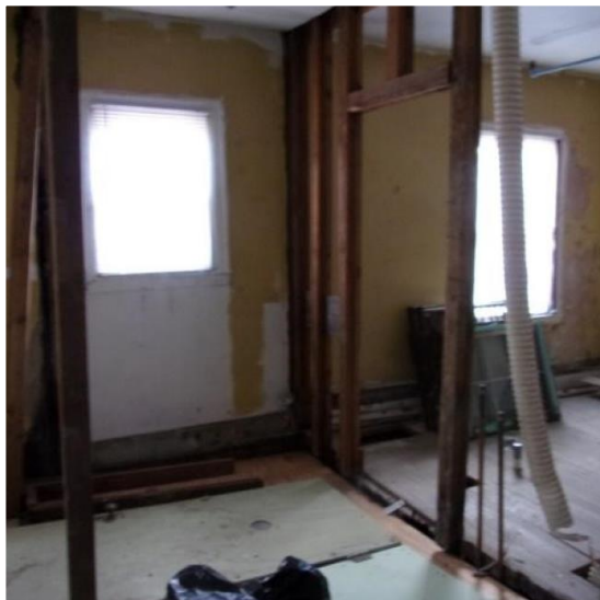
3rd Floor Under Renovation
