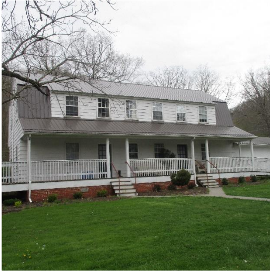
3rd Structure Looking West
