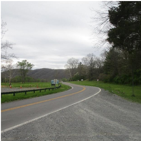
Street Scene Looking East Back to Subject
