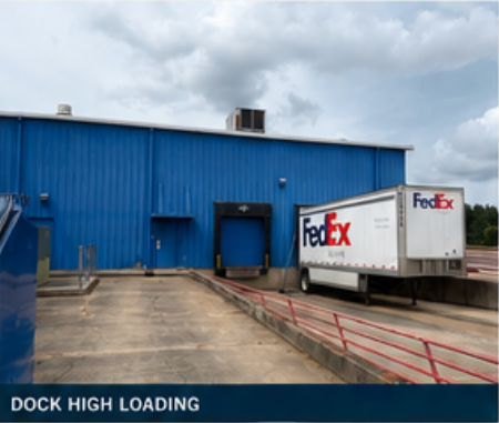
DOCK HIGH LOADING
