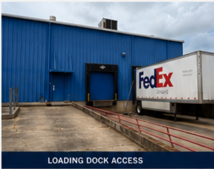
LOADING DOCK ACCESS
