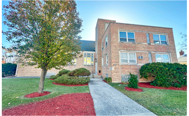
SIDE OF BUILDING
