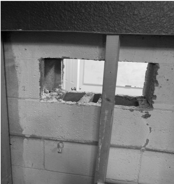
West Wall Removal Location
