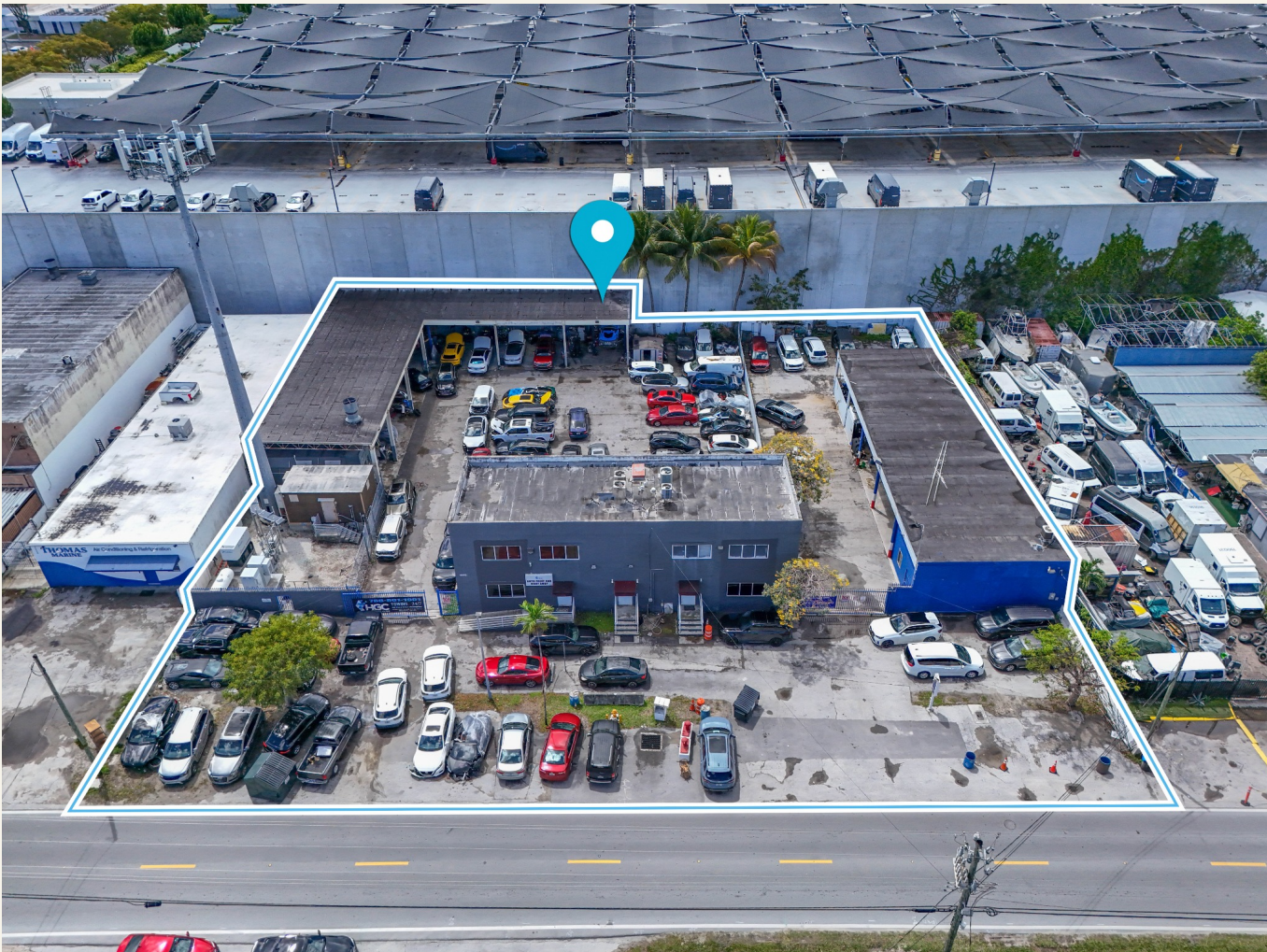
Aerial view of 3326 NW South River Drive, outlined in blue — two-story operations building, one-story storage building, and paved yard with dedicated collision-shop circulation.
