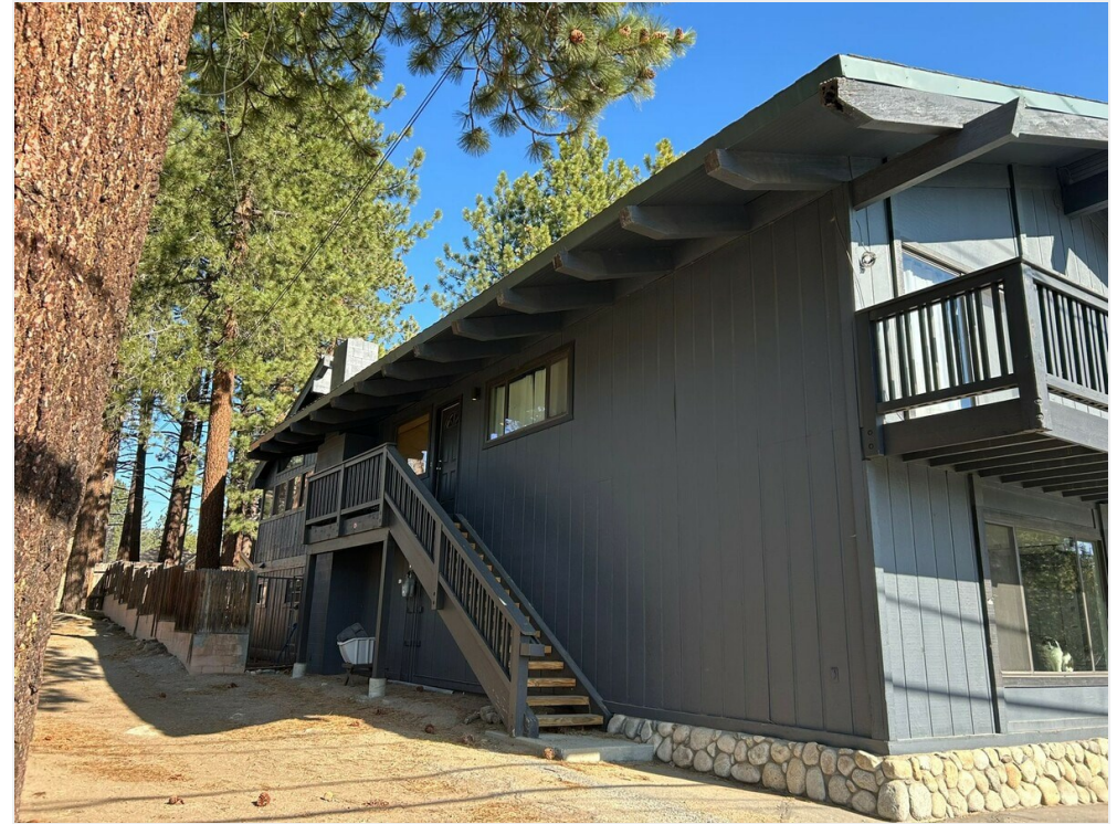
38 LMT Side Apartment Stairs Entrance
