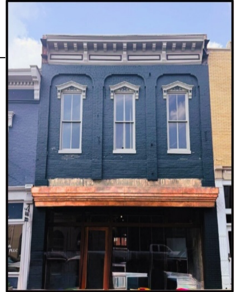
Exterior: Main Street Façade
