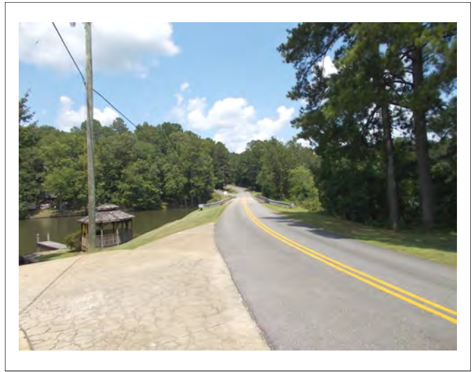
Barrons Bridge Road facing northeast. View from the drive of the subject property
