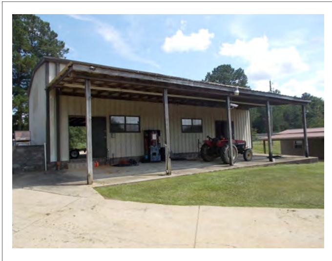
Workshop located on the subject property near Barrons Bridge Road
