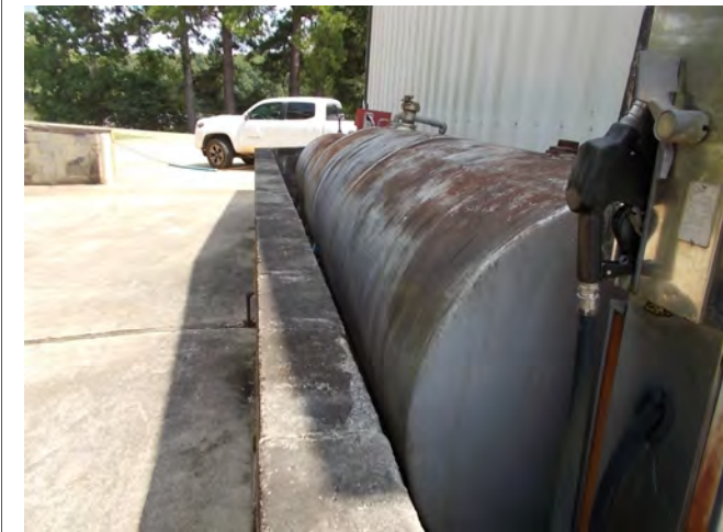
Two above ground storage (AST) containing ethanol free gas present on the subject property. The eastern and western tanks have a capacity of 500 gallons and 1,000 gallons respectively
