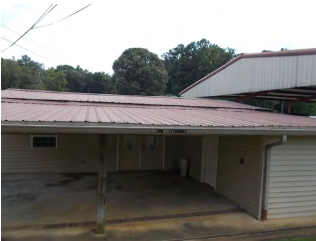
Storage building present along the southeastern boundary of the subject property.
