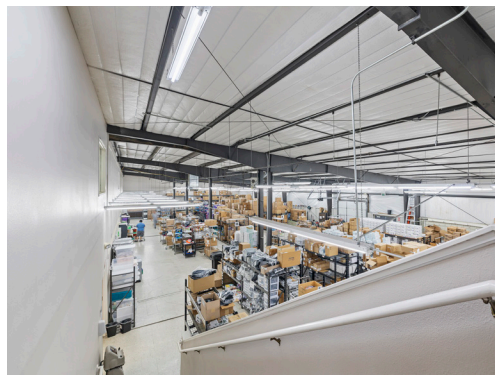
View of Warehouse from Second Floor Offices
