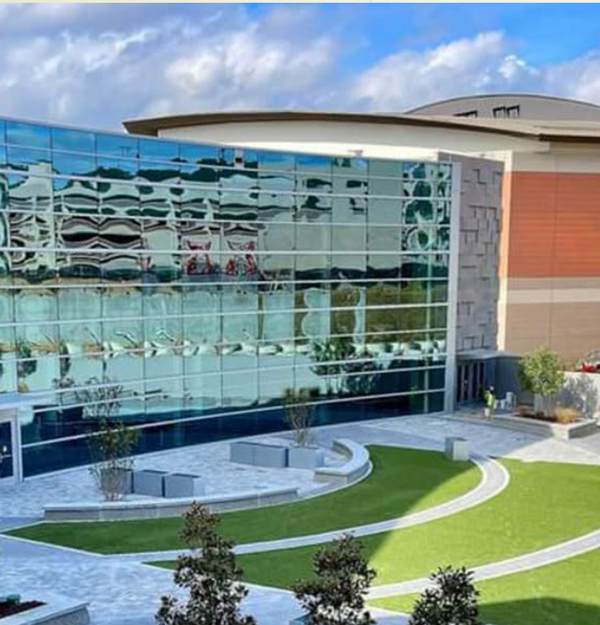
GAS SOUTH CONVENTION CENTER
