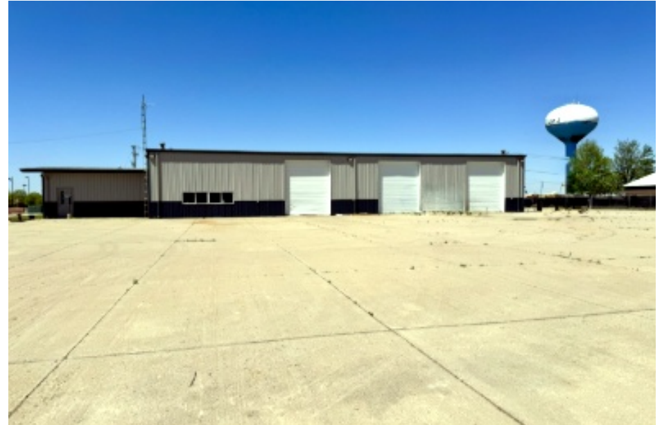
Multiple Overhead Doors with Large Concrete Yard
