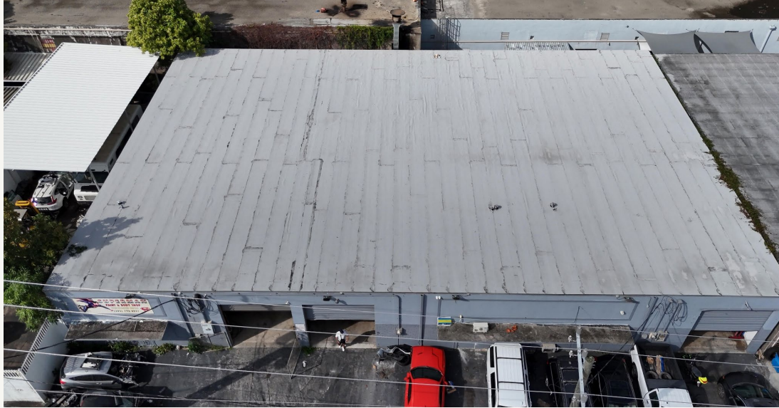
Roof recovered in 2022, per ownership
