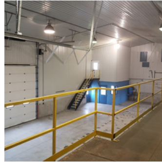
Mezzanine with 2nd floor Storage for Parts/Tires
