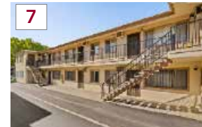
7 437 W GLENOAKS BLVD GLENDALE, CA 91201
