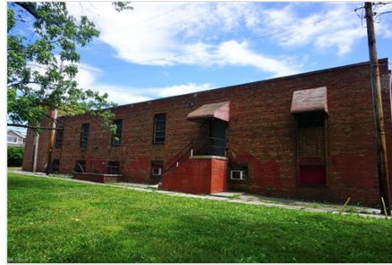
W. Side of building
