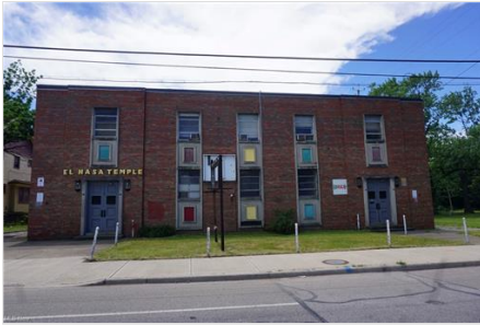
Solid brick building
