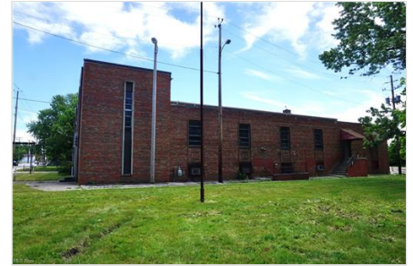
W. side of building
